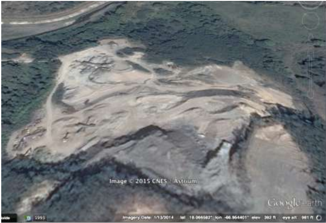
Figure 16. Typical quarry occurring on slopes with no visible sediment control basins or ponds.
