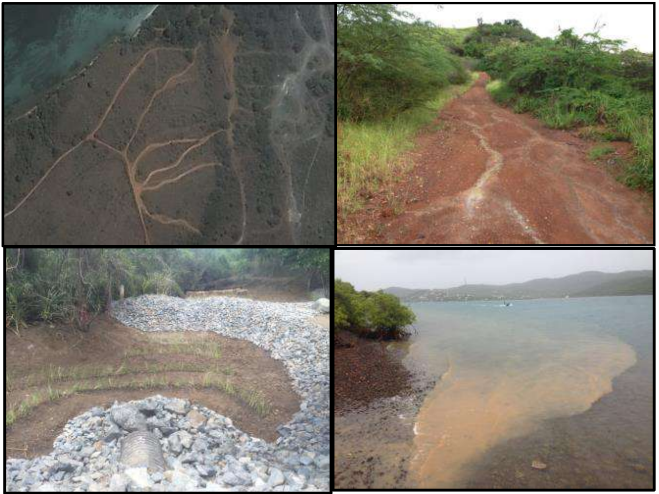
Figure 13. Clockwise from top left: Dirt roads in Los Pozos near Combate, a significant source of sediment to coastal waters, (right) example of surface rills conveyance over the road surface creating erosion and resulting in fine sediment losses, bottom right sediment reaching coastal waters; bottom left: recently constructed sediment trap in Cabo Rojo to capture sediment before it enters Boquerón Bay
