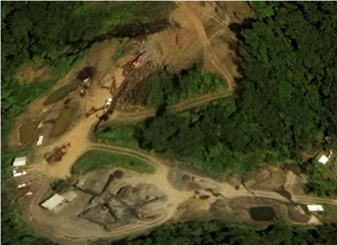
Figure 17. Quarry sediment basin (in lower right of photo) for a project in Faga'alu, American Samoa
