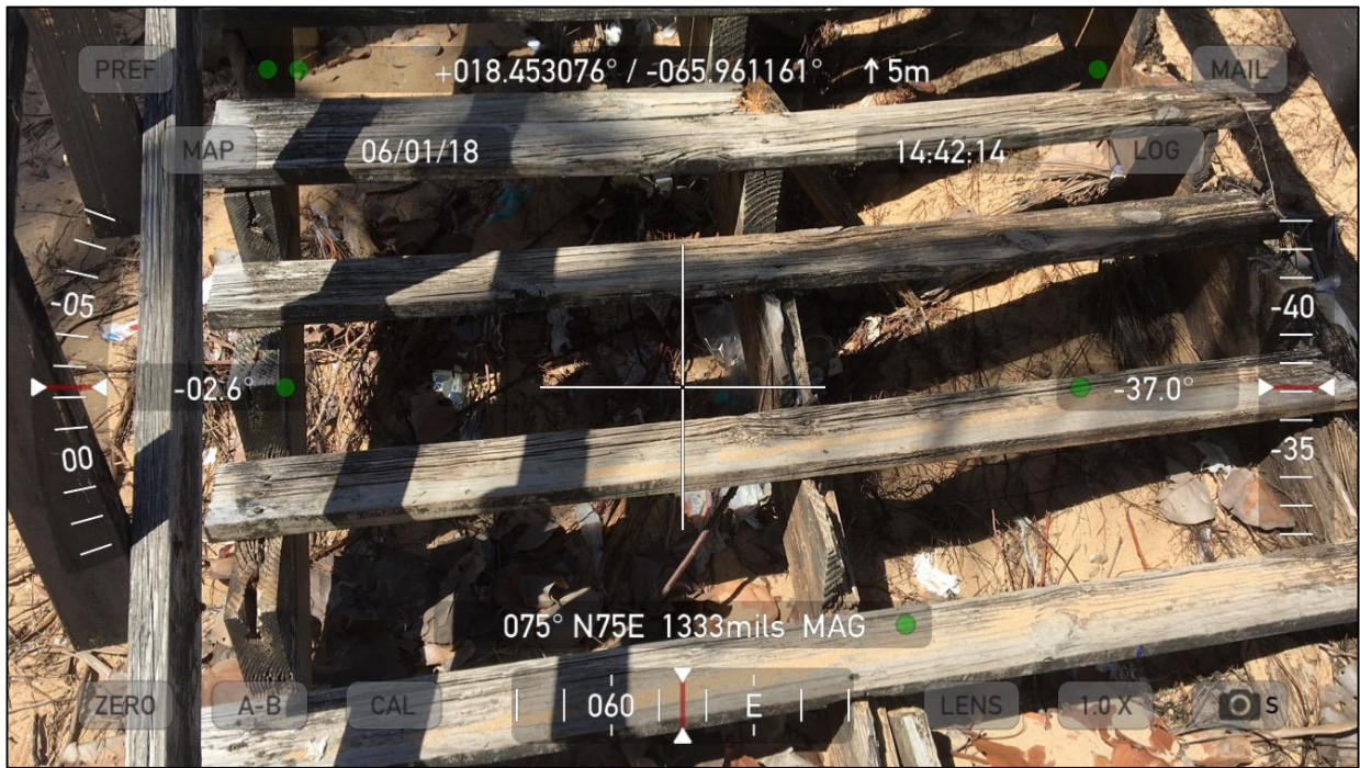
Figure 7. One of the wooden boardwalks on the primary dune along PR-187.
