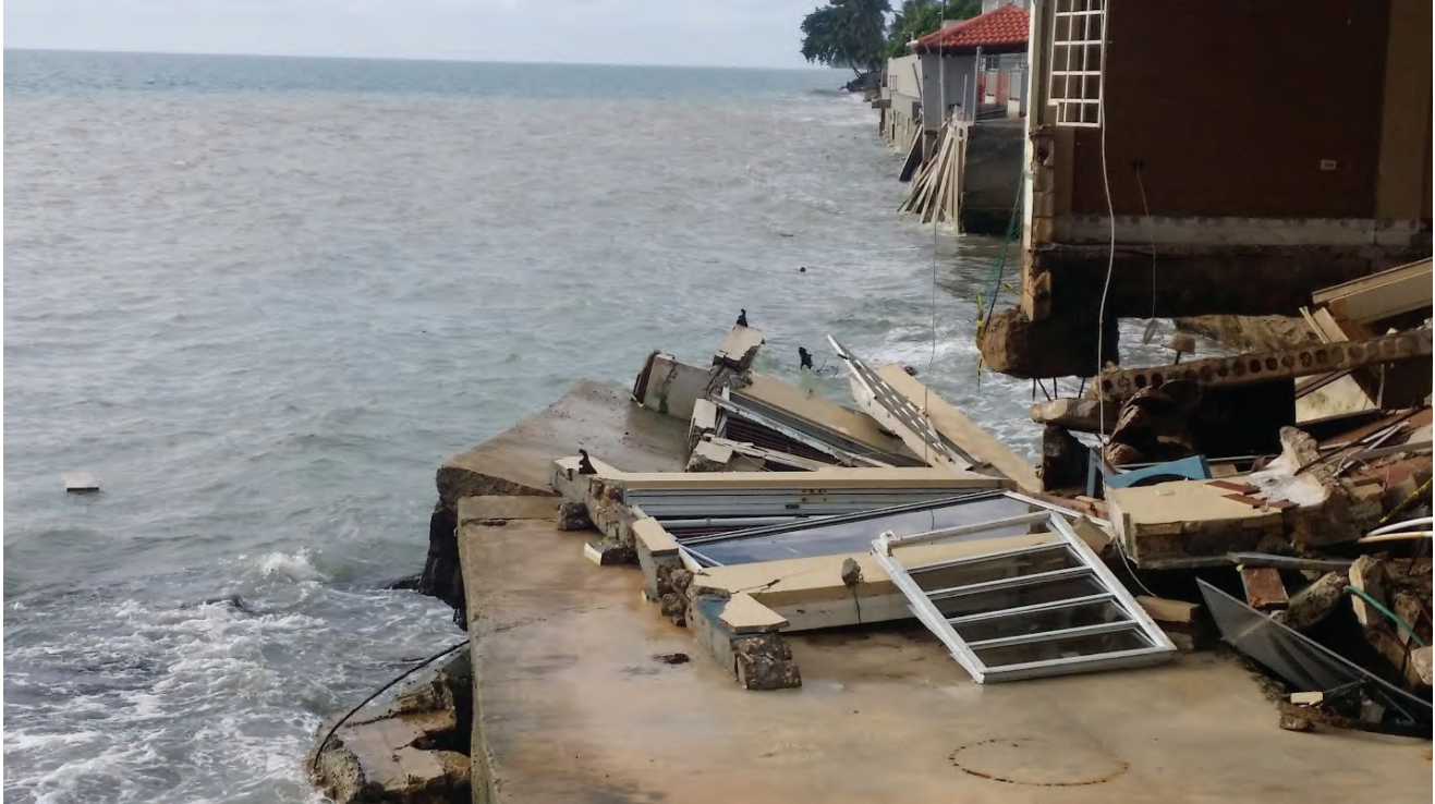
Catastrophic failure of unprotected waterfront properties at Rincon. Photo: DNER
