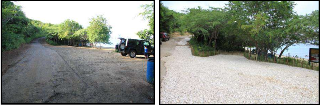
Figure 17. Before and after stabilization at Tamarindo Beach in Culebra
