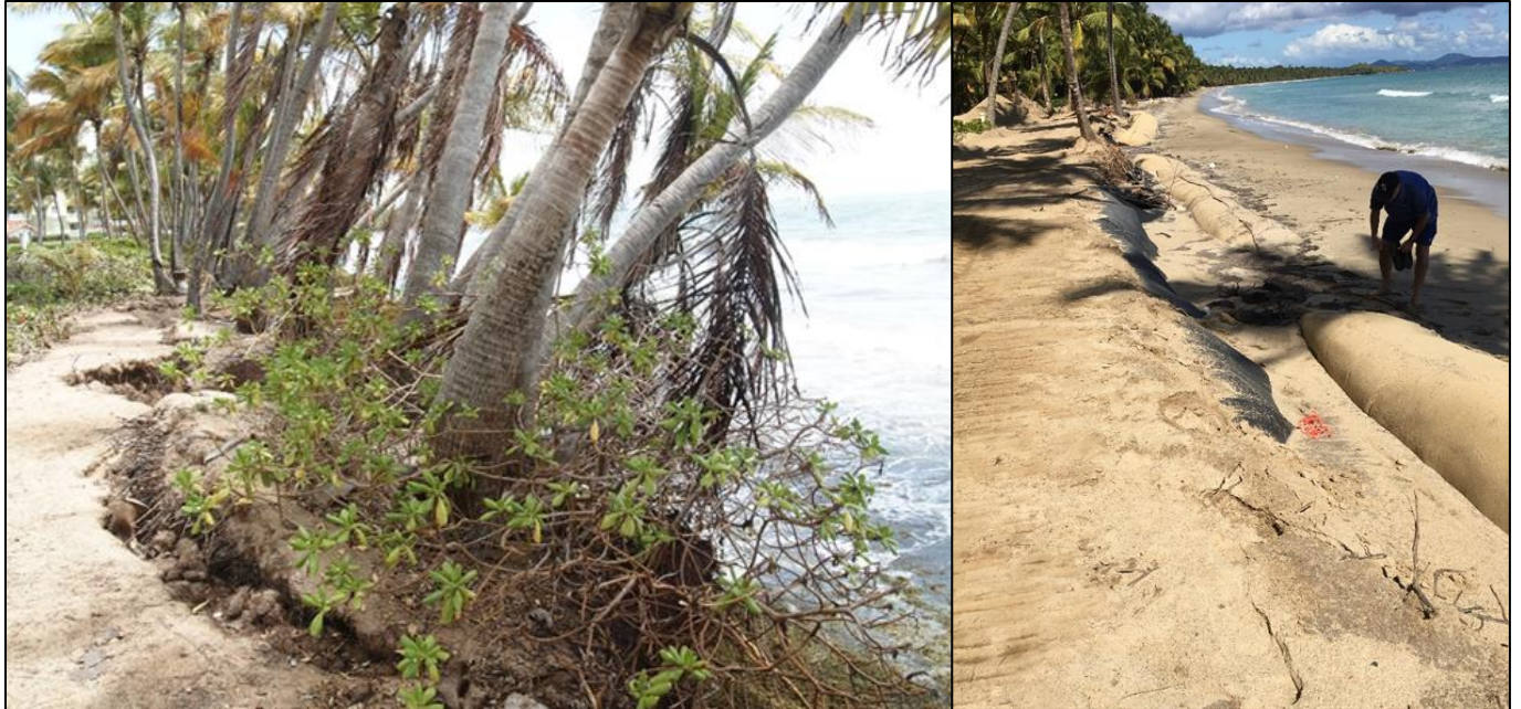
Figure 18. An eroding shoreline at Marbella Club, Palmas del Mar (left photo). Sand filled geotubes were placed along the shoreline in January 2016.
