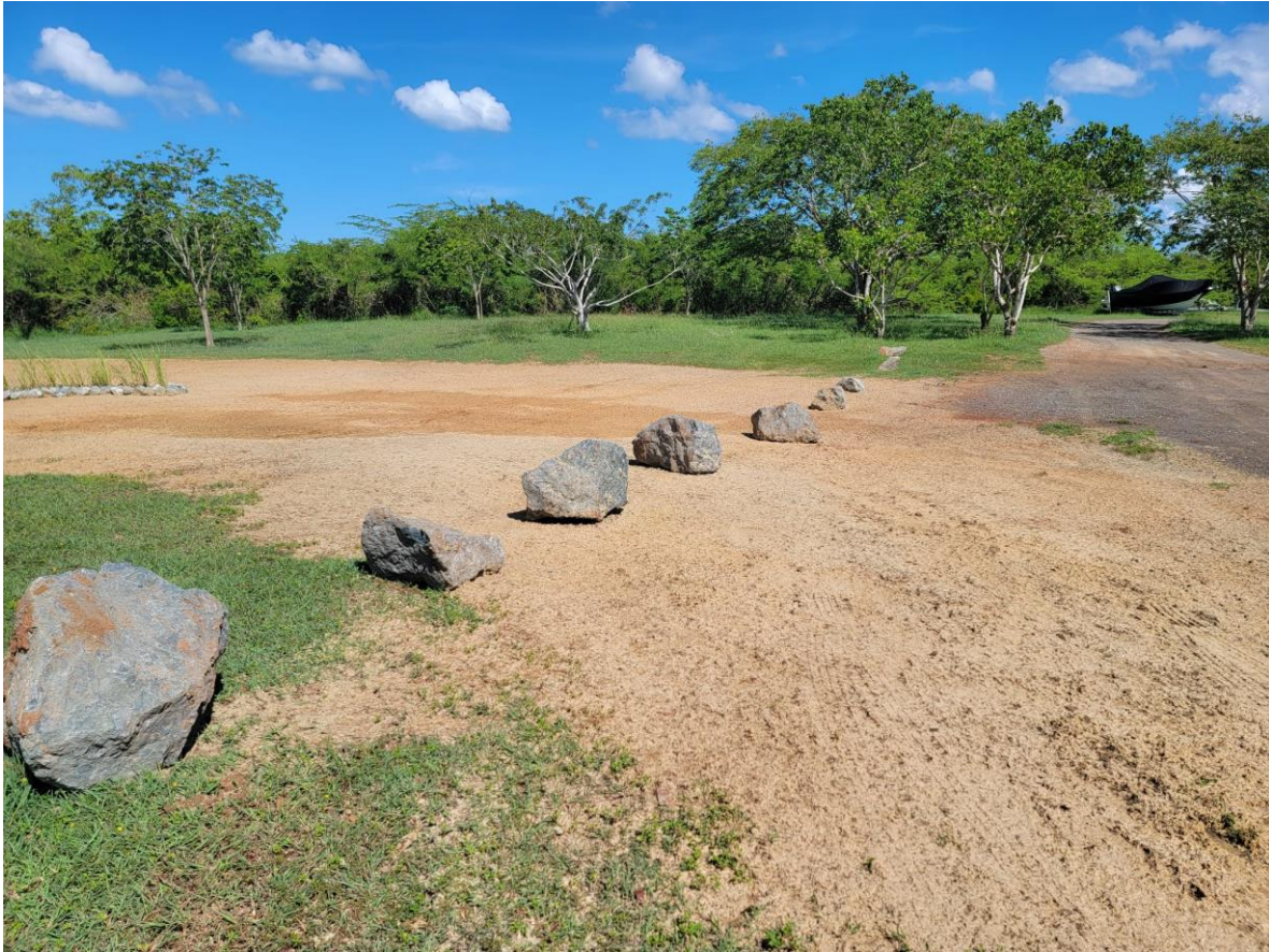
Image 18. The project team installed rocks to prevent cars from entering and damaging the rain garden.
