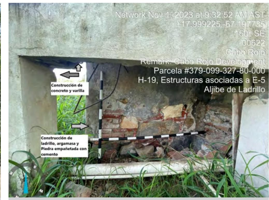
H-19 - ESTRUCTURA DE CONCRETO Y LADRILLO
